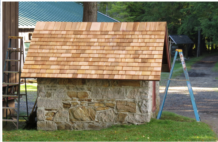
The smoke hosue at Camp Huntington gets a new roof
